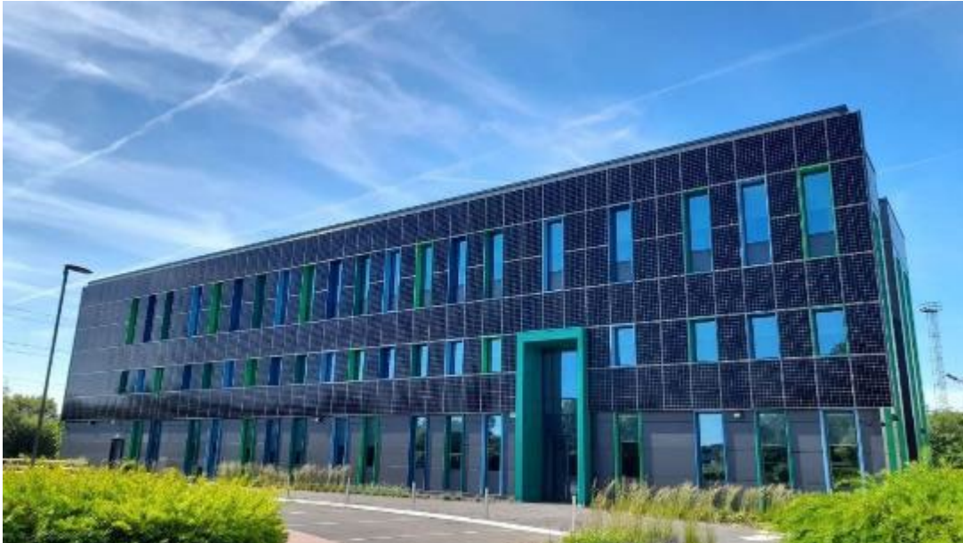
Figure 6: The Bay Technology Centre – Groundbreaking & multi award winning operational energy positive building for commercial use
