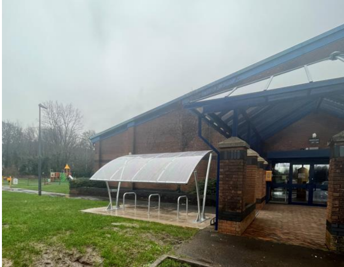
Figure 8: Picture showing cycle storage installed at Vale of Neath Leisure Centre.
