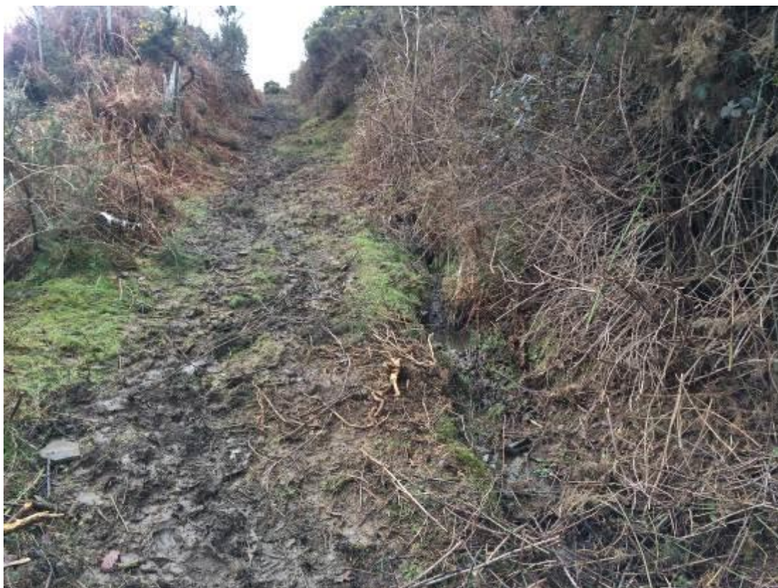
Photograph 18 – Small issue of water alongside access track
