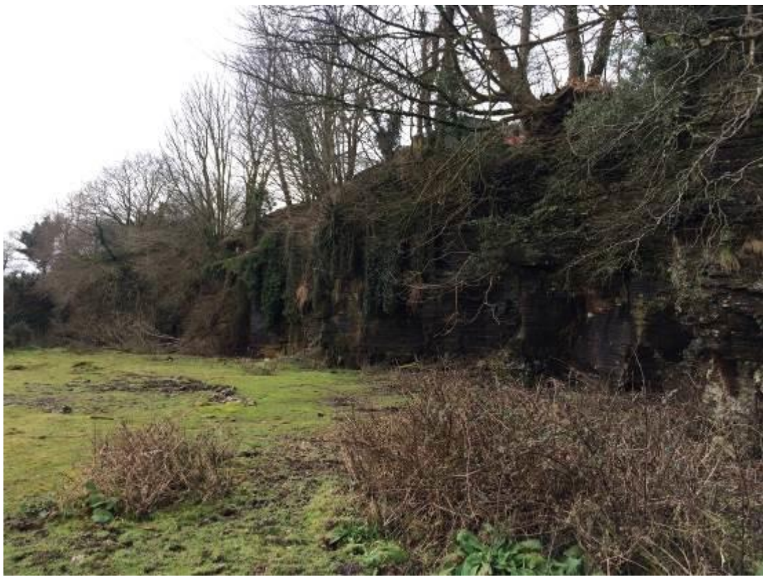
Photograph 4 – Quarry high wall showing vertical face
