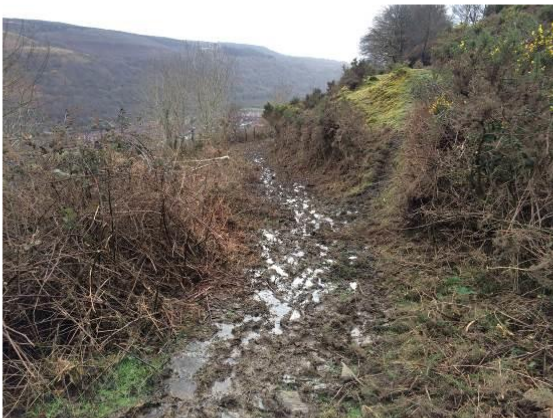
Photograph 19 – Water flowing along route of access track
