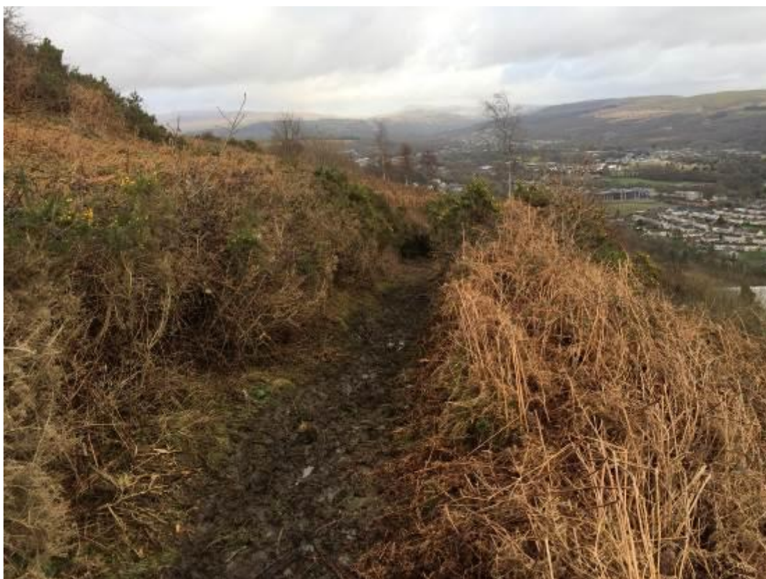
Photograph 17 – Access track cleared to lower bench
