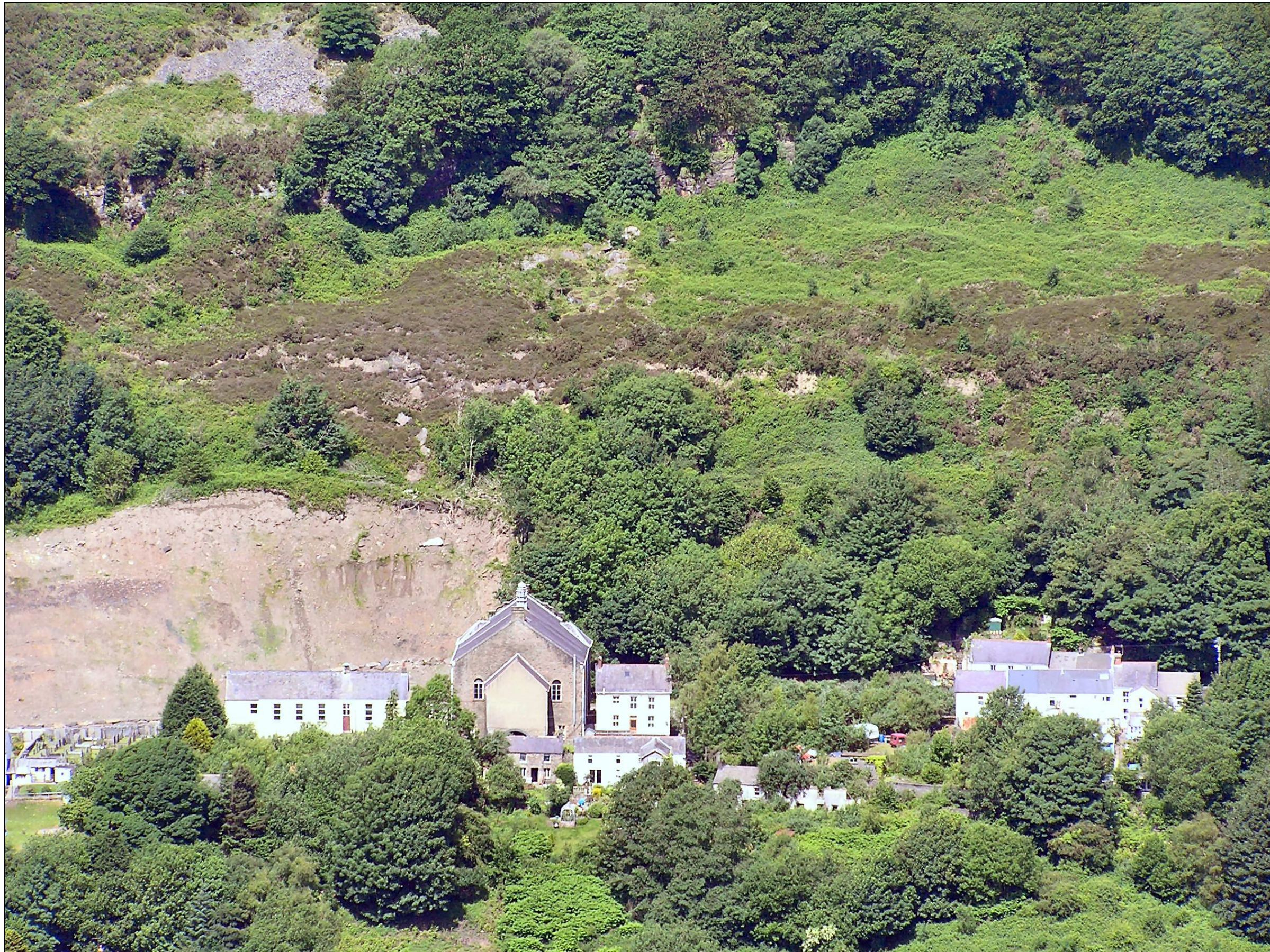
Plate B-6: Pantteg Landslip area, showing extent of the fissuring on the hillside above the 2013 regrading.
