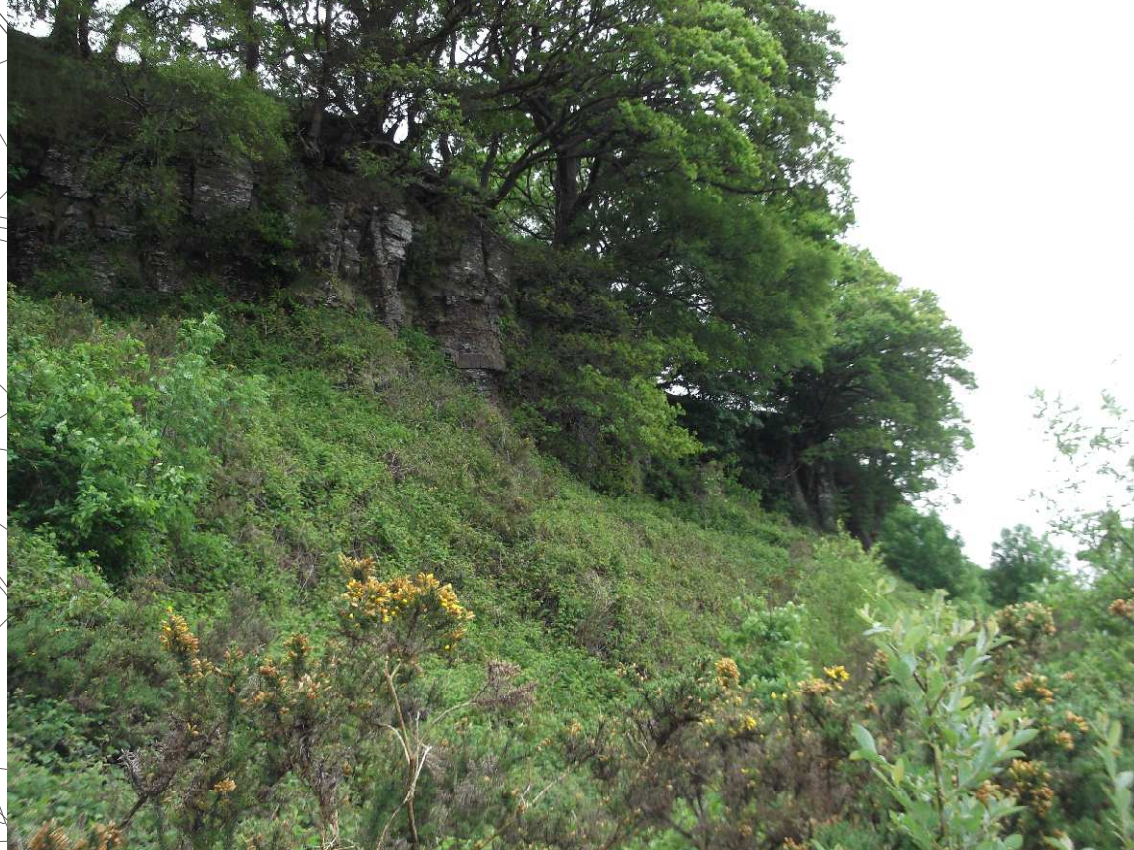
CLIFFS OF LLYNFI ROCK SANDSTONE AT BACKSCARP OF PANTTEG LANDSLIP
