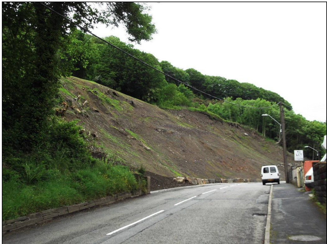
Plate A-6: Pantteg – regraded slope from the south-west.
