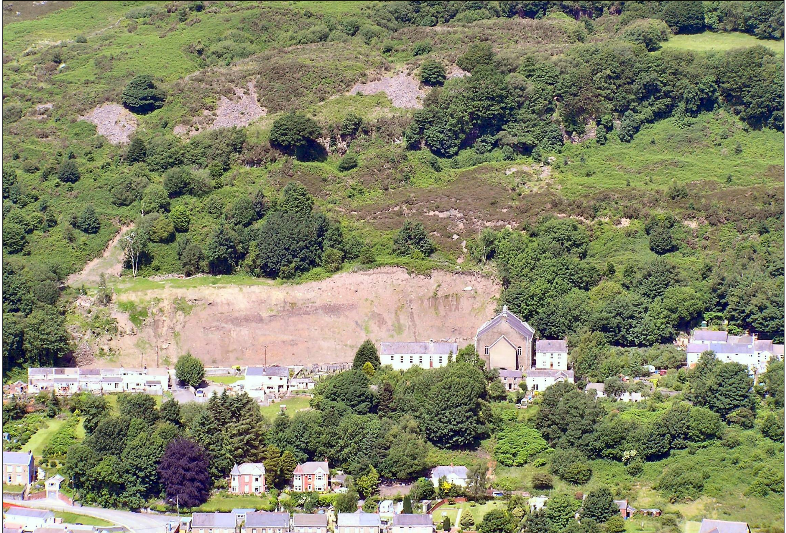
Plate B-5: Pantteg Landslip area, showing extent of 2013 regrading works.
