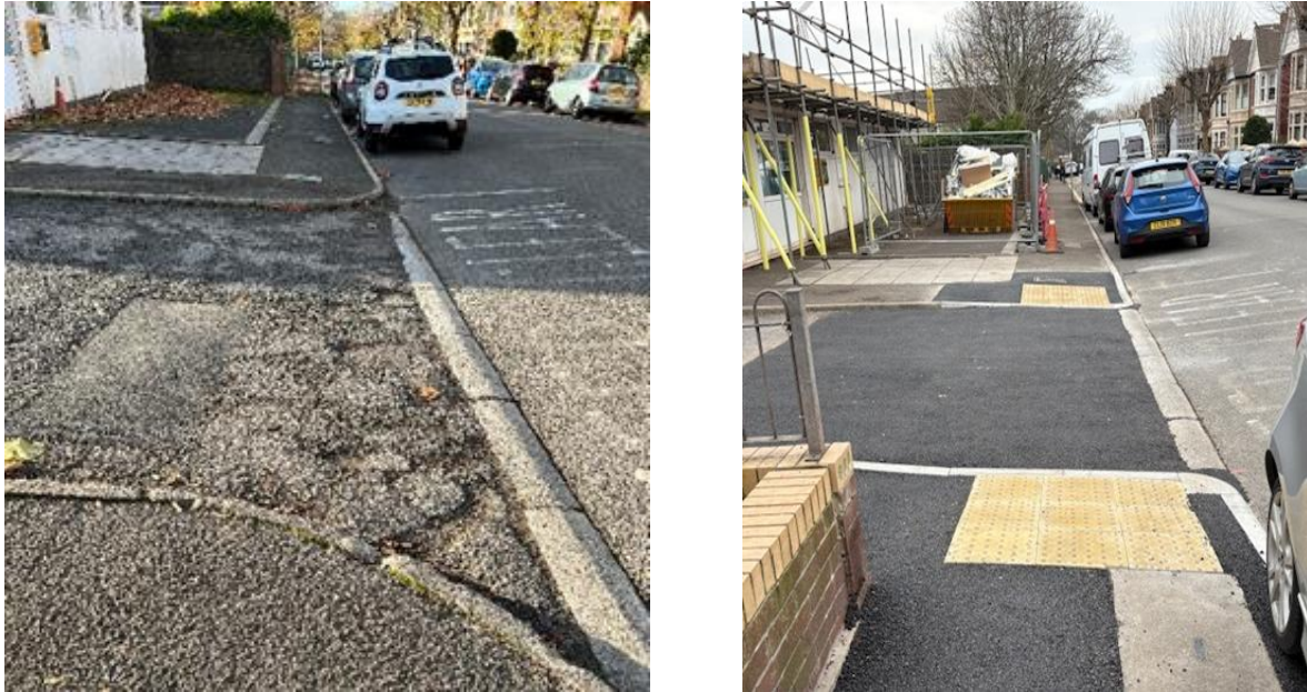
Figure 5: Example of a before and after photo of a new dropped kerb/tactiles on Theodore Road, Port Talbot
