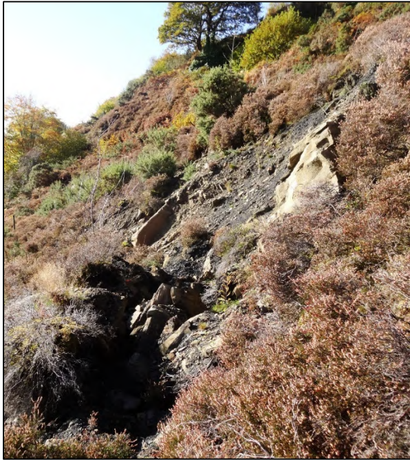
Insert 3 - Photograph of tension cracking on the break of slope above Pantteg Chapel exposing boulders of Llynfi Sandstone. Aerial photographic interpretation has identified several landslides to occur along this break in slope. Hazard Type 2 and 6. Photograph taken 28 th October 2015 looking south-west
