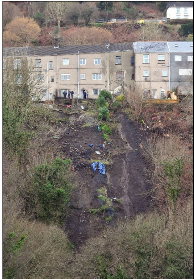
Insert 39 - 2017 landslide at rear of No. 86 Cyfyng Road http://www.walesonline.co.uk/news/wales-news/homes-evacuated-after-swanssea-valley-12680597
