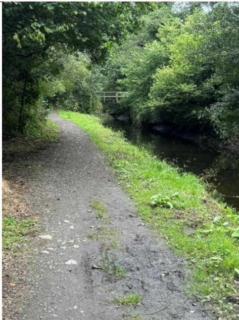
Image 67 – Section of Neath Canal with trees overhanging
