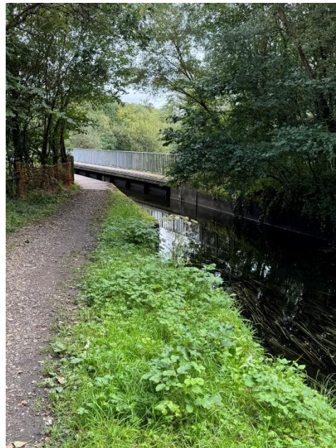
Image 68 – Ynysbwlllog Aqueduct with well- maintained footpath
