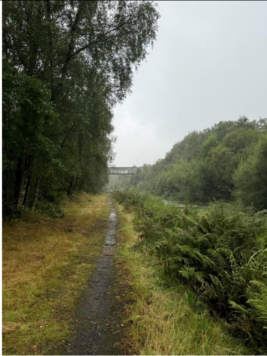
Image 37 – Gas works bridge with narrow footpath
