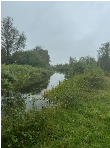
Image 43 - Jersey Marine Bridge canal section in moderately good condition
