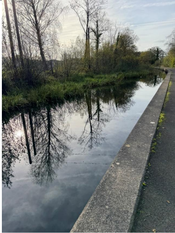
Image 22 – Canal in good condition near Link Road Bridge
