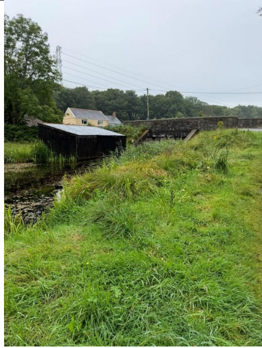
Image 42 – Jersey Marine Bridge with grassy shrubs surrounding
