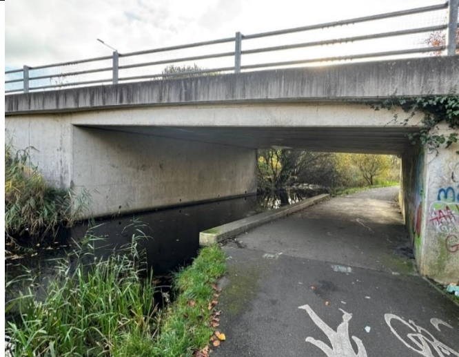
Image 14 – Metal box Bridge with pedestrian and cycle path
