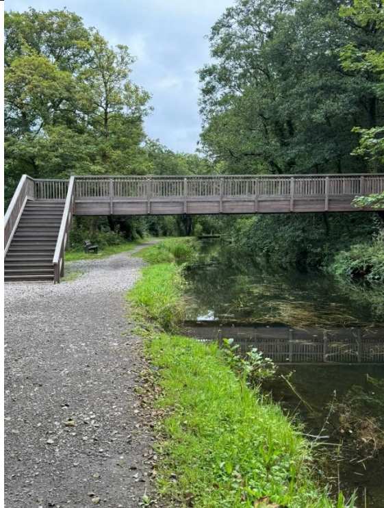
Image 42 – Howards Footbridge over Neath Canal
