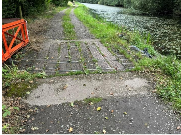
Image 58 – Spillway in footpath to River Neath near Ynysnedd Bridge
