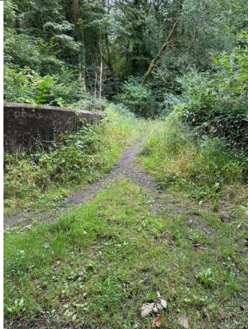
Image 48 – Pontygwaith Bridge path
