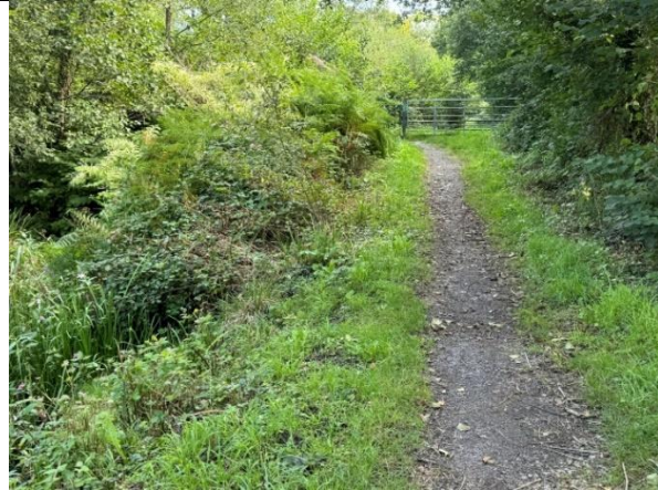
Image 74 - Ynysarwed Isaf Lock currently inoperable
