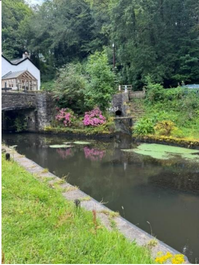
Image 37 – Tonna Lock Structure viewed from opposite embankment
