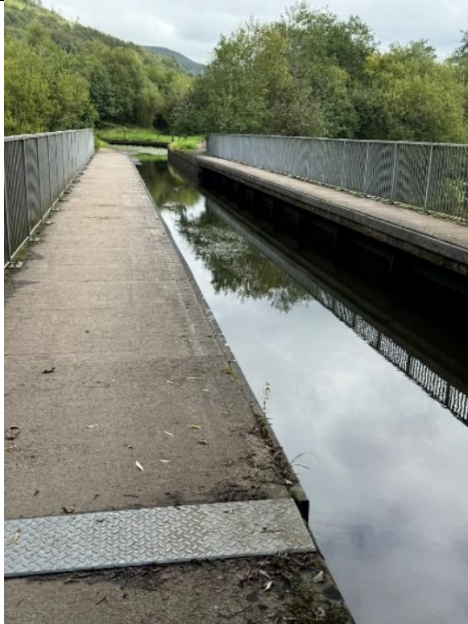
Image 69 – Ynysbwlllog Aqueduct in well maintained condition
