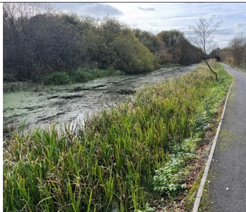
Image 11 – Pipe Bridge with some vegetation on side bank with path in good condition
