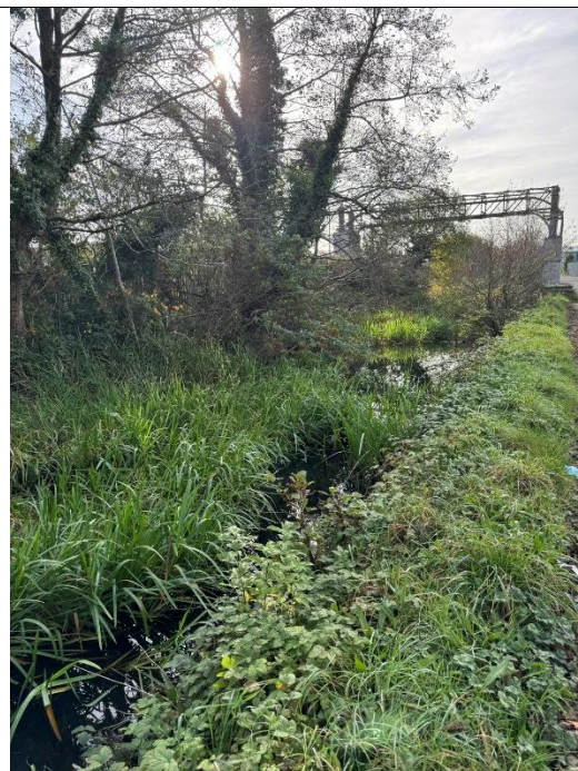
Image 28 – Pipe bridge with surrounding truss structure and overgrown canal
