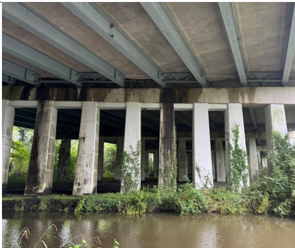
Image 35 – M4 Bridge with canal adjacent to bridge
