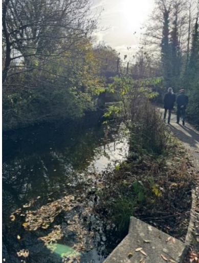
Image 23 – Section of the canal near Link Road Bridge with light vegetation on banks
