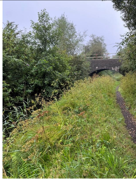
Image 30 – Crown Copperworks Bridge
