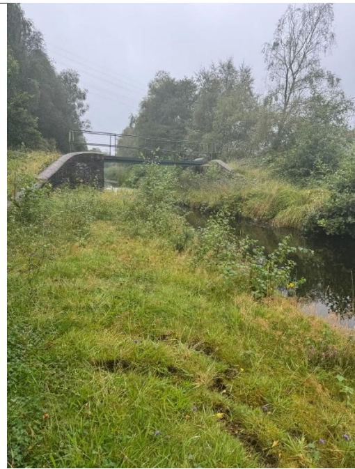
Image 40 – Quarry Bridge with shrubs on embankments
