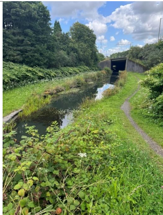
Image 4 – Overhead Roundabout/viaduct/bridge on A465
