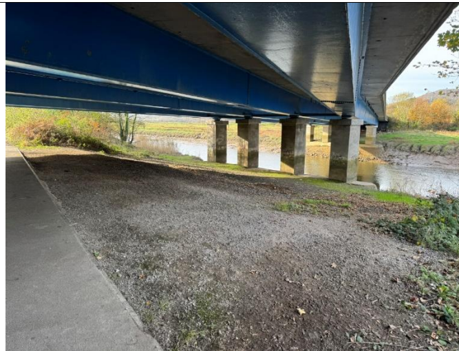
Image 20 – Link Road Bridge
