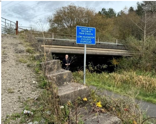
Image 7 – Landfill Site Bridge with low headroom but sufficient for canal
