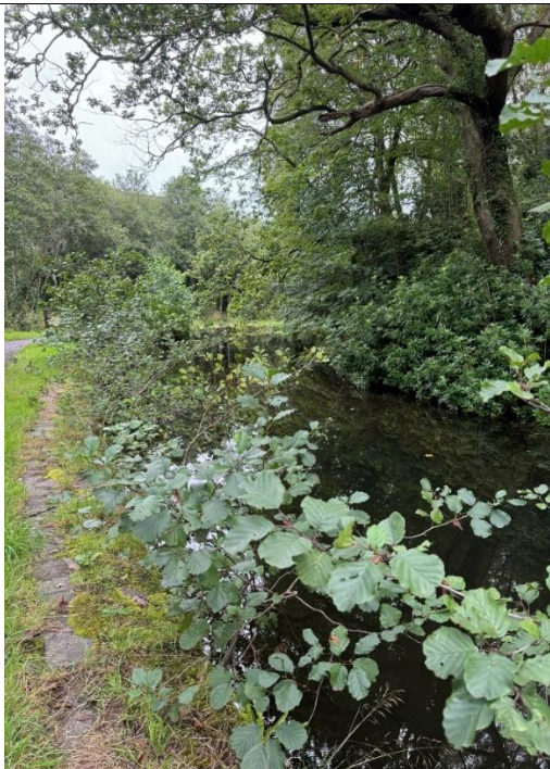
Image 43 – Trees and bushes growing on canal embankments near Howards Footbridge
