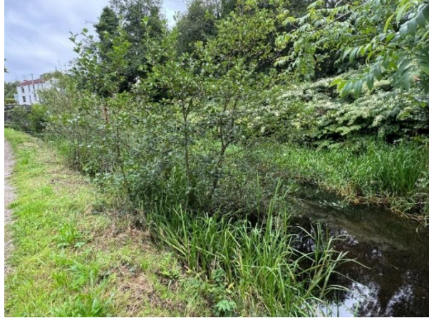
Image 62 – Reeds/shrubs clogging canal near Abertwrch Bridge
