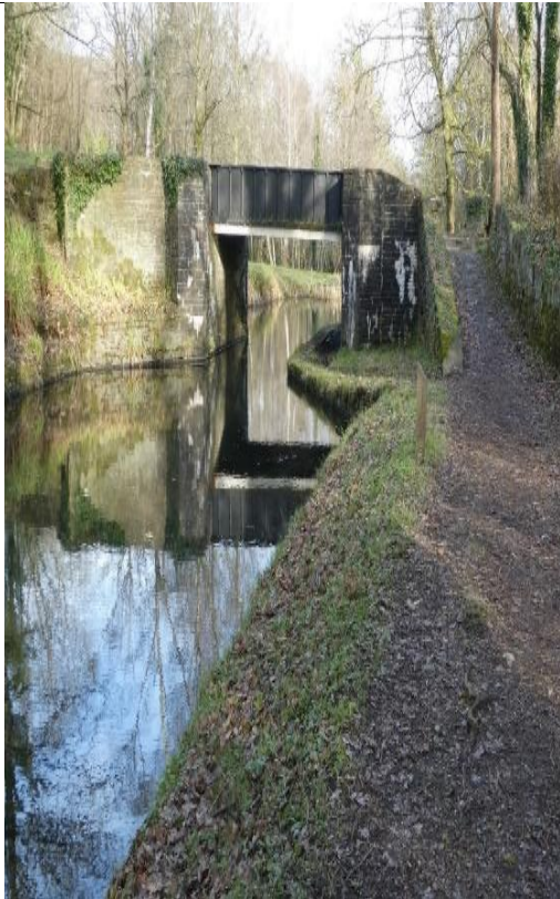
Image 83 – Rheola Iron Aqueduct
