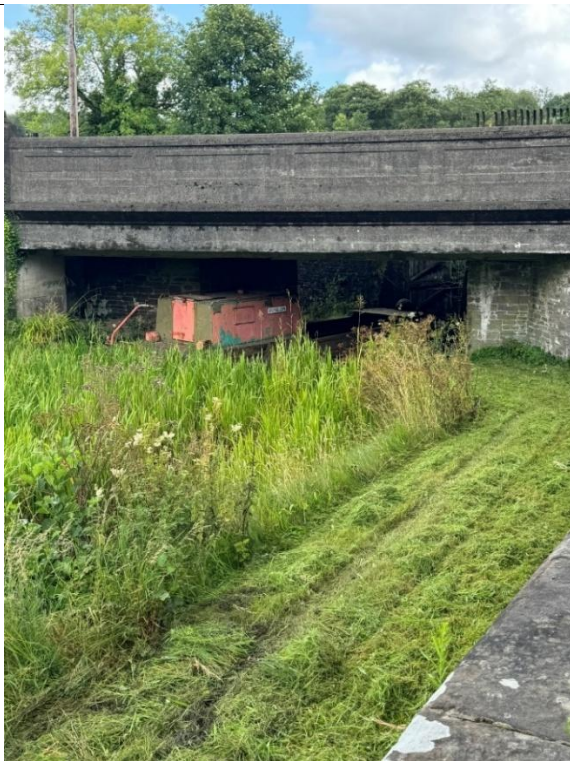
Image 3 – Station Road Bridge
