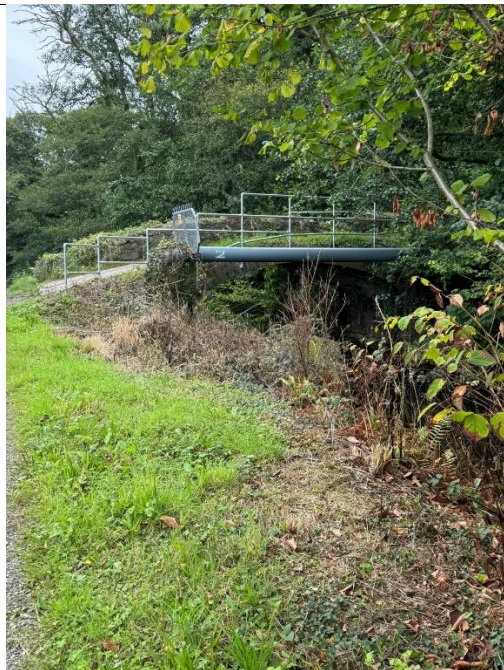
Image 55 – Ynysnedd Bridge with adjacent pipe bridge
