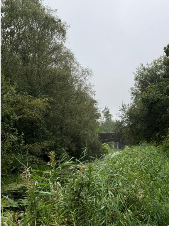
Image 26– Skewen Tramroad bridge
