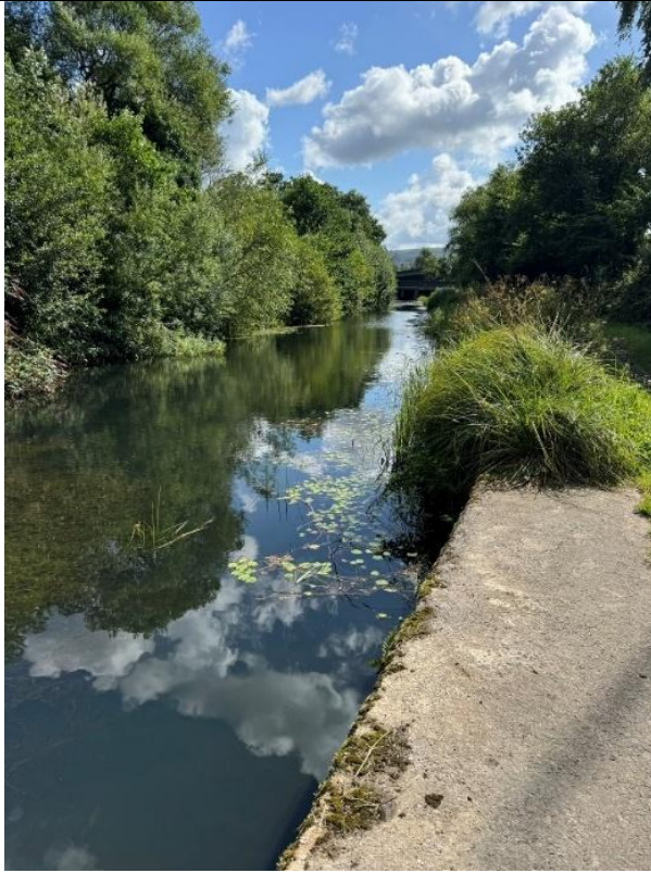
Image 17 – A465 bridge approach canal section
