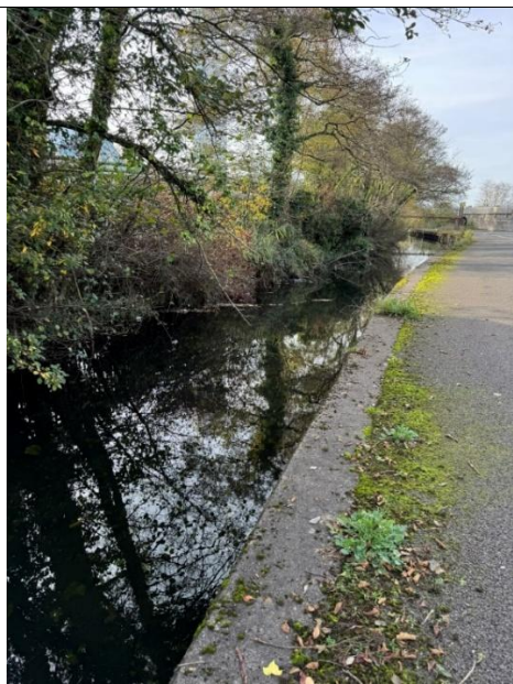
Image 27 – Canal section near Milland Road Bridge with trees overhanging
