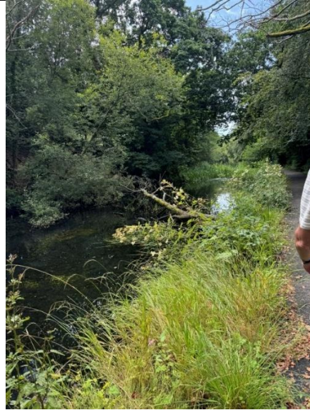
Image 34 – Canalside bridge with low vegetation on embankment
