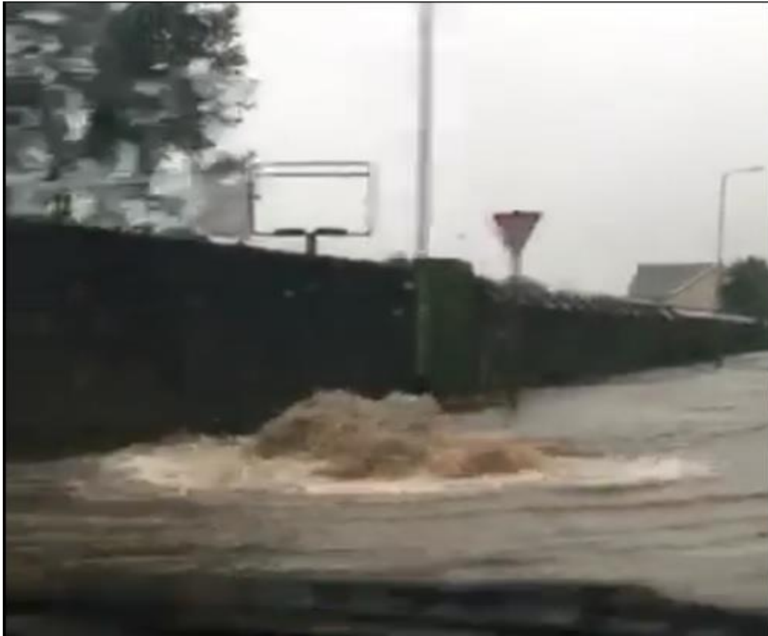
Figure 9, Picture showing surcharging water from Ynysydarren culvert
