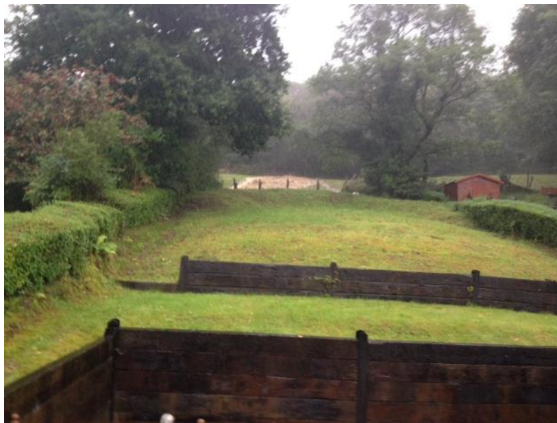
Figure 8, Culvert intake structure (ID: CUL_0432) during flood event
