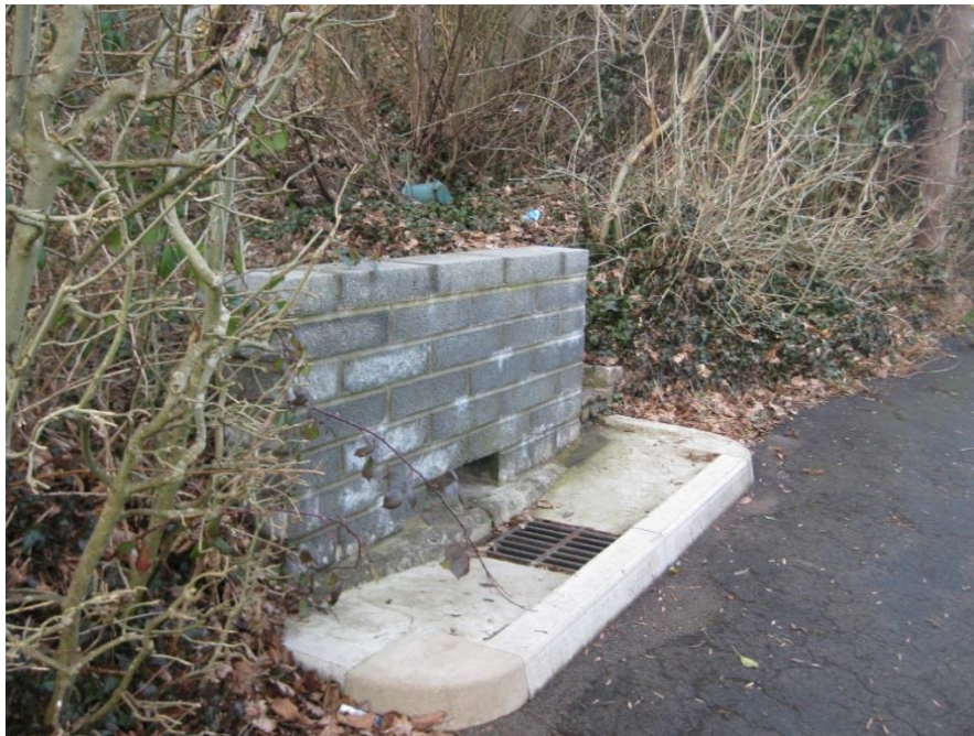
Figure 6, Culvert intake structure (ID: CUL_0186)
