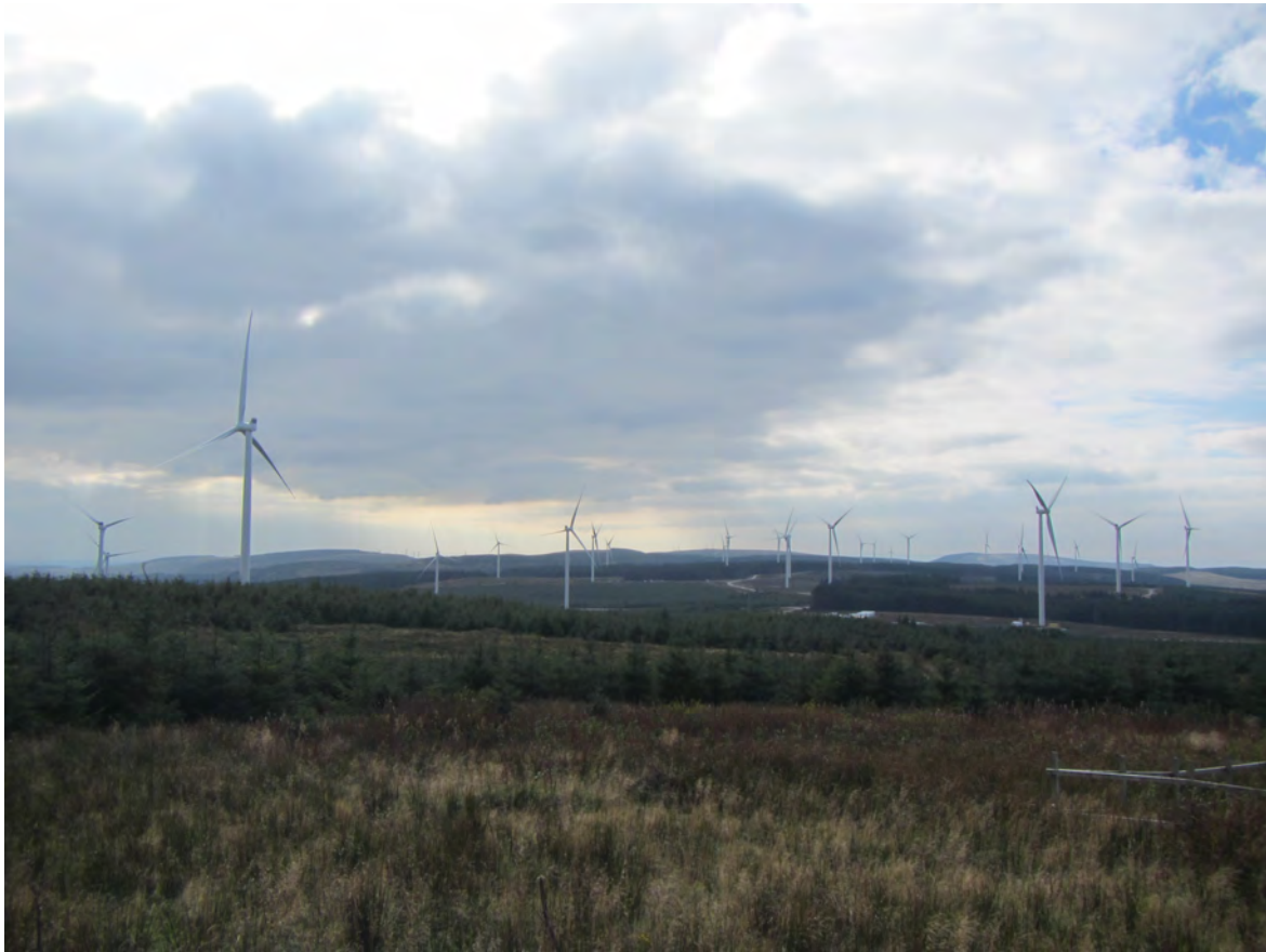
Picture C.1 Wind Turbines at Pen y Cymoedd Wind Farm
