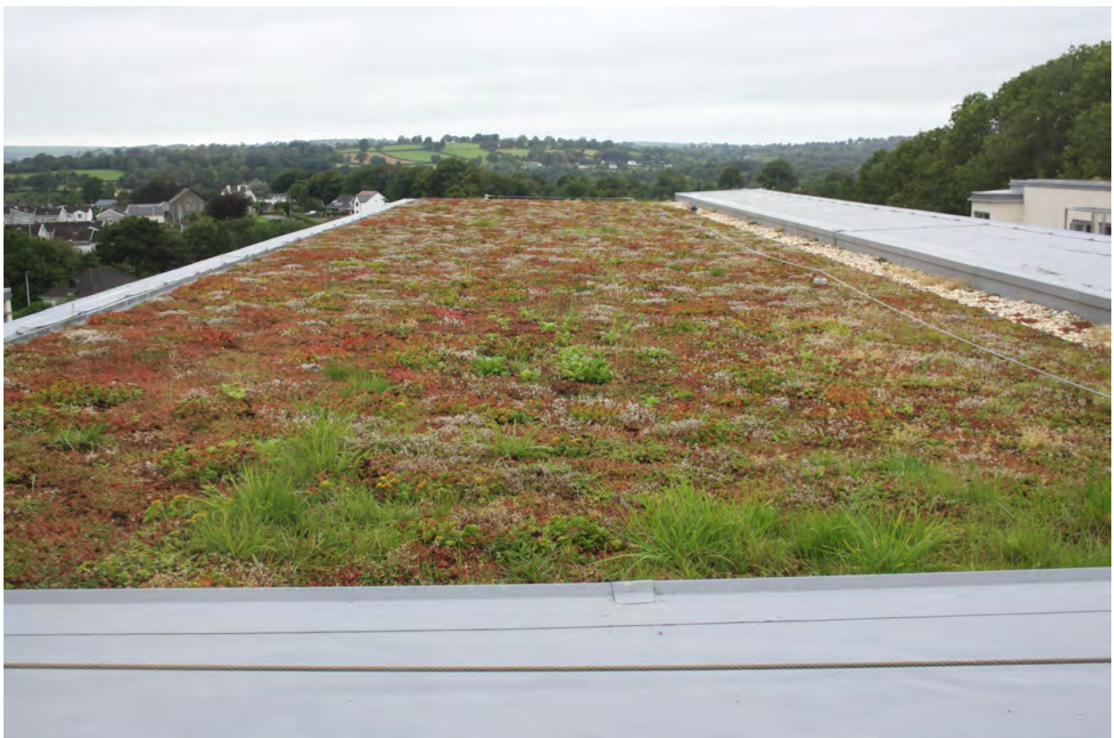
Picture 5.4 Living Roof (Copyright Chris Jones)
