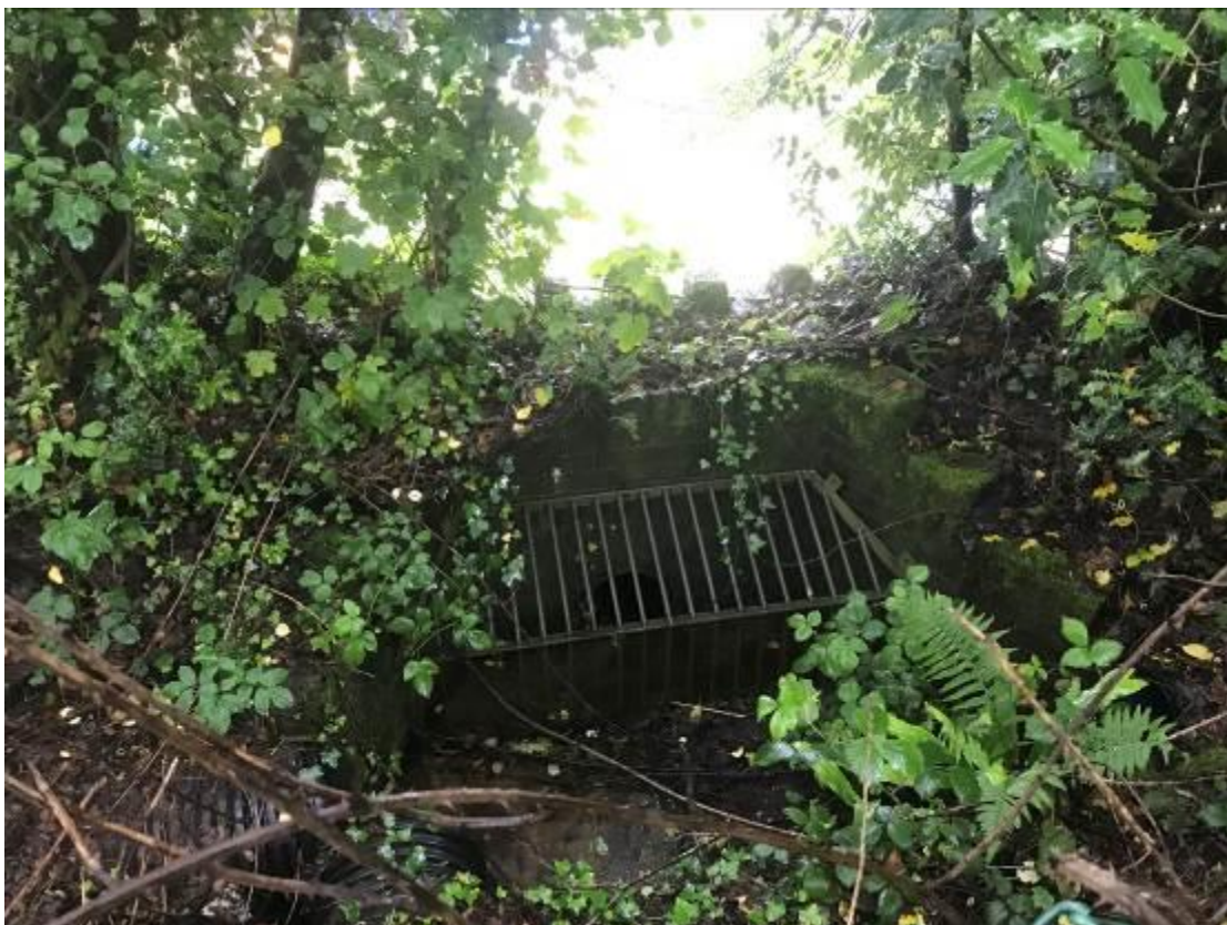
Photograph 36 – Inlet chamber at rear of school
