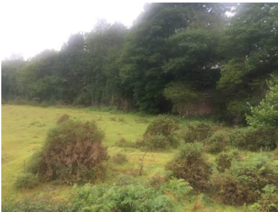
Photograph 1 – Quarry high wall location
