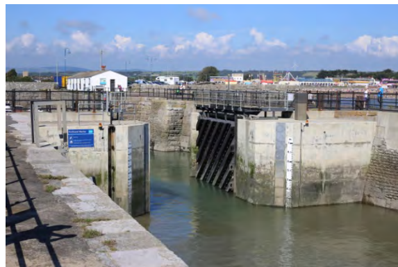
The harbour entrance with new lock gates
