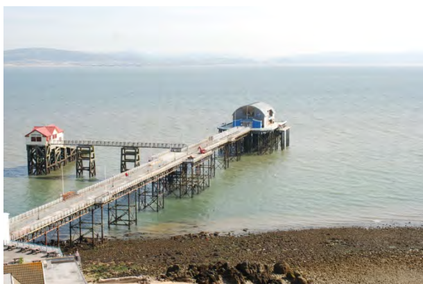
The old and new life boat stations at Mumbles Pier form landmarks at the western end of the bay and are an indication of the use of the water over the years
