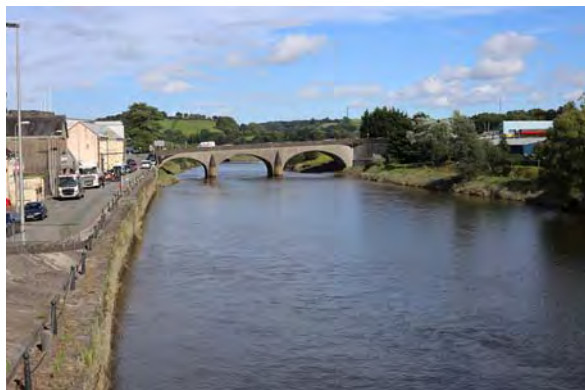
The tidal river bridge at Carmarthen
