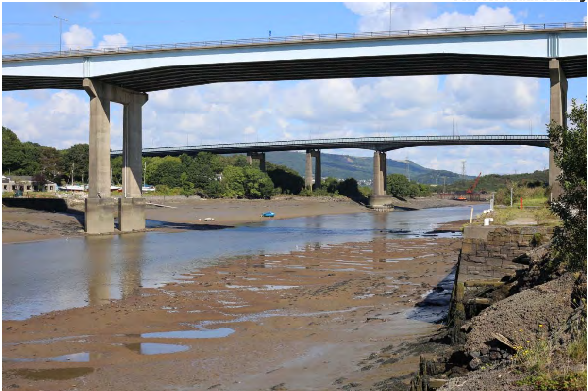
The Neath/Nedd estuary at low tide running beneath the M4 and A48 bridges looking towards Giant's Grave wharf
