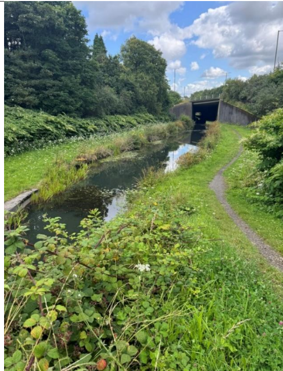
Image 8 – Vale of Neath Railway Canal section in relatively good condition
