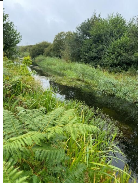
Image 44 – Access Road canal section with reeds on both embankments
