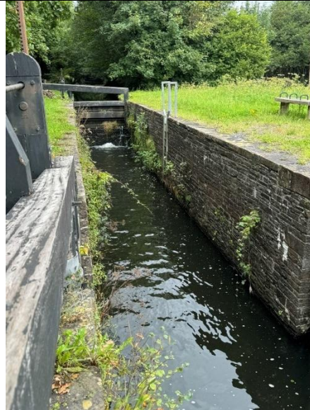
Image 64 – Clun Isaf Lock currently inoperable with view of access ladder
