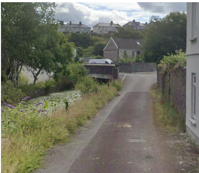
Figure 7-10 - Diamond Bridge Briton Ferry
