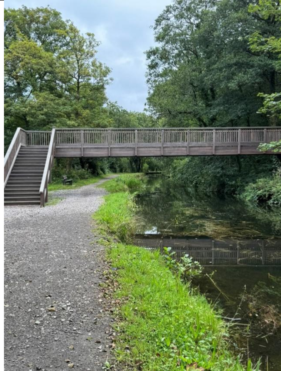
Image 42 – Howards Footbridge over Neath Canal
