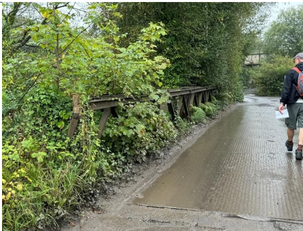
Image 31 – Abbey Wharf Bridge
