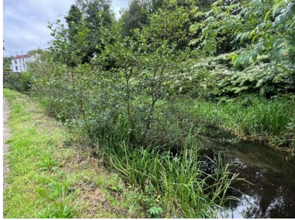
Image 62 – Reeds/shrubs clogging canal near Abertwrch Bridge
