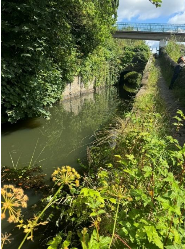
Image 13 – Bridge Street Bridge
