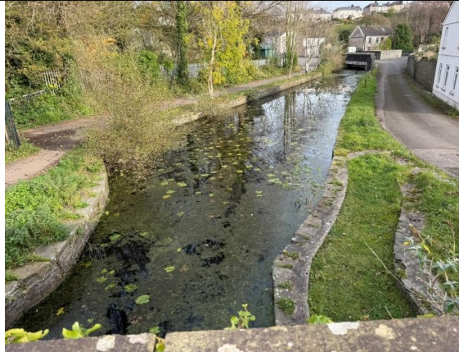
Image 2 – Canal viewed from Diamond Bridge showcasing structure and canal condition
