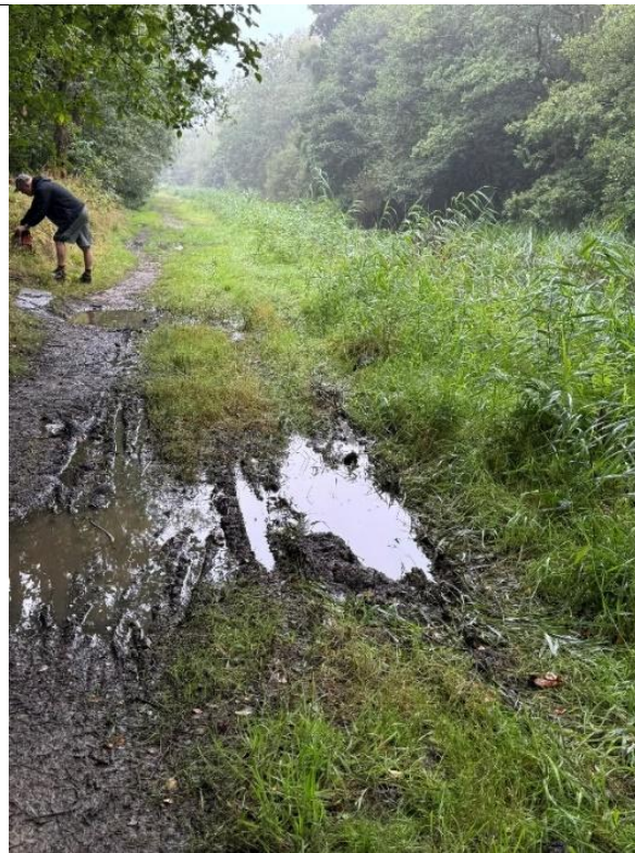
Image 36 – M4 Bridge canal section with minor footpath flooding
