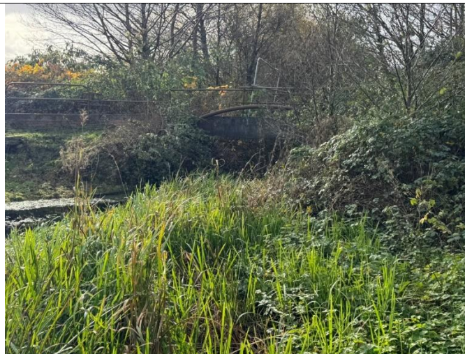
Image 12 – Tricks Bridge structure partially hidden by thick vegetation
