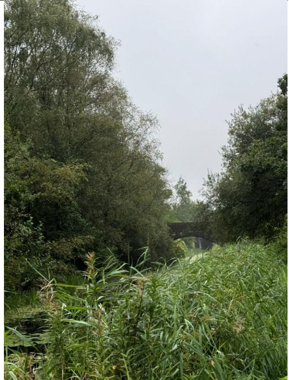
Image 26– Skewen Tramroad bridge
