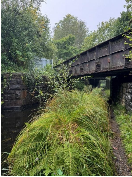
Image 41 – Rhondda and Swansea Railway Bridge with narrow footpath
