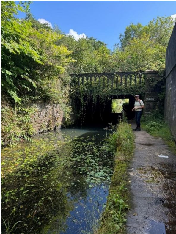
Image 7 – Vale of Neath Railway Bridge
