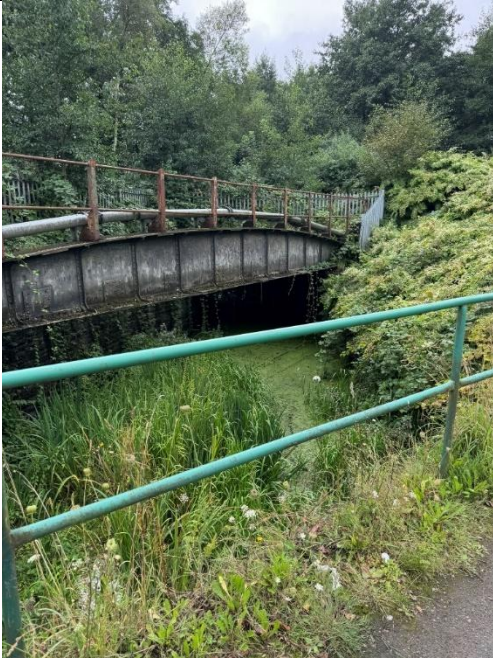
Image 45 – Former Vale of Neath Railway Bridge
