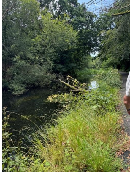
Image 34 – Canalside bridge with low vegetation on embankment
