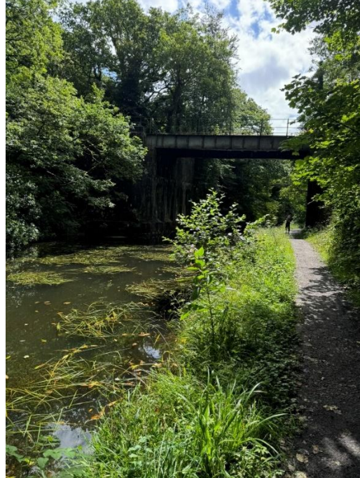
Image 40 – Vale of Neath Railway Bridge over canal
