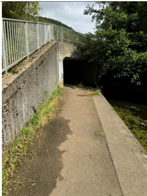
Image 71 – A465 Bridge with pedestrian footpath adjacent to canal
