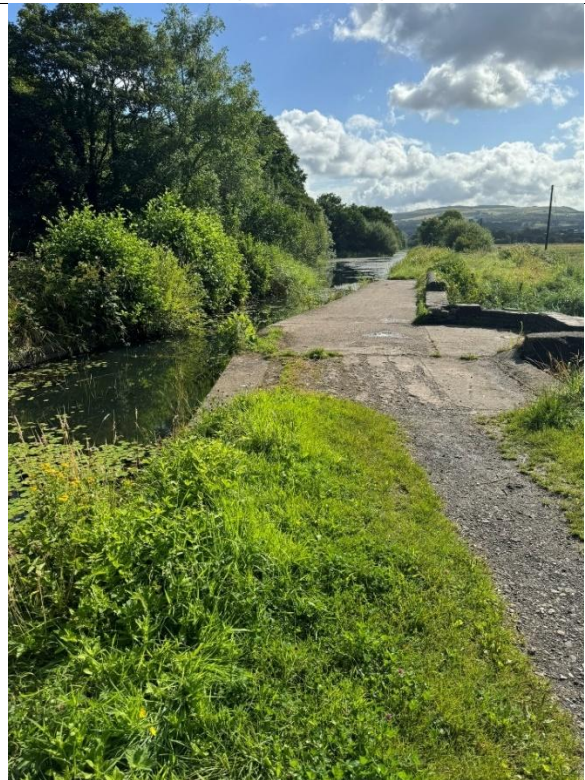
Image 20 – Spillway into River Neath
