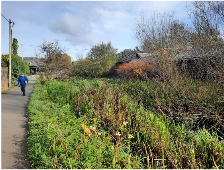
Figure 7-8 - Channel between Bridge Street and Milland Road Bridges
