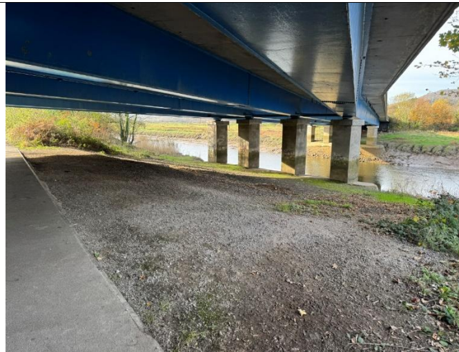
Image 20 – Link Road Bridge
