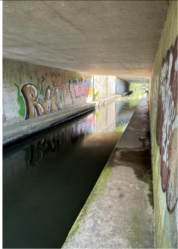
Image 18 – A465 approach bridge with narrow pedestrian path
