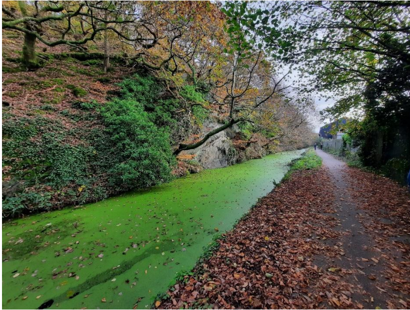
Figure 7-11 - Channel section between Diamond Bridge and River Neath
