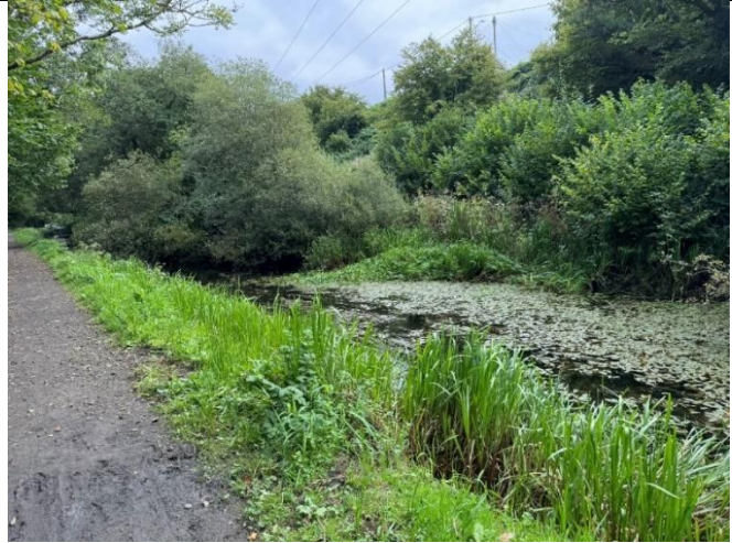
Image 70 – Section of the canal near Ynysbwlllog Aqueduct with reeds and lily pads obstructing navigation
