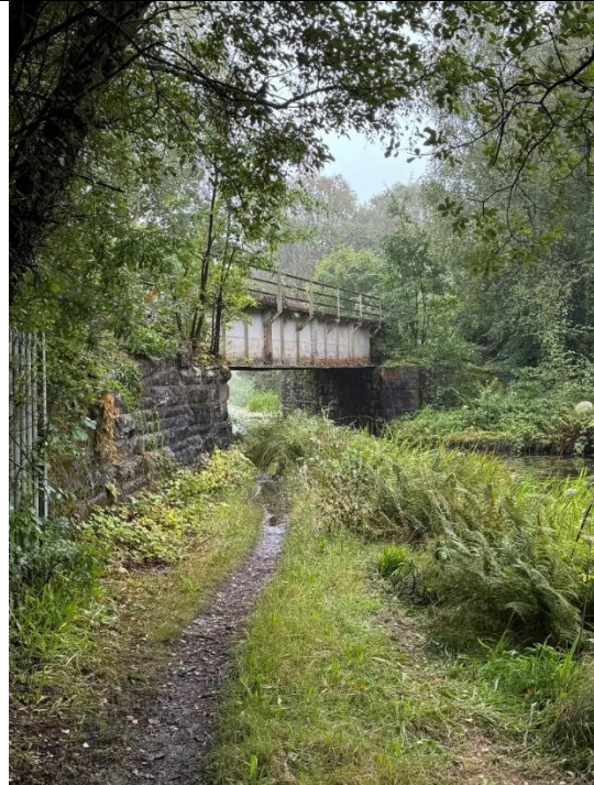
Image 38 – Railway Bridge with narrow footpath
