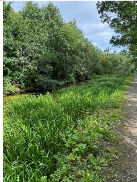
Image 76 – Canal clogged with reeds near Ynysarwed Isaf Lock
