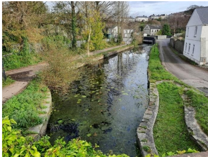
Figure 10-14 - Diamond Bridge Terminus
