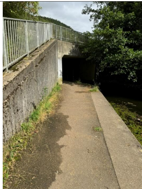
Image 72 – Ynysbwlllog bridge with light vegetation on footpath
