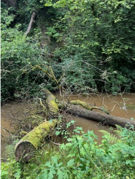
Image 39 – Canal section near Dulais Fach Road Bridge with fallen tree in canal
