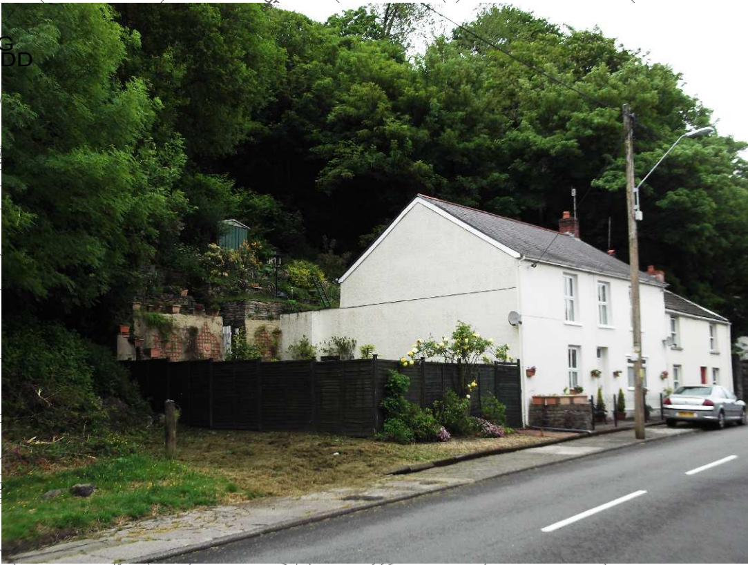
21-27 PANTTEG, SHOWING PROXIMITY OF SLOPE TO REAR OF PROPERTIES
