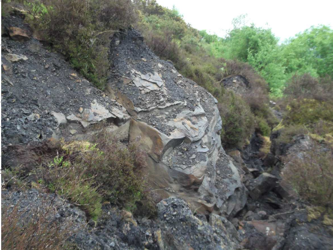
FISSURES IN TERRACE ABOVE 2012 FAILURE AREA
