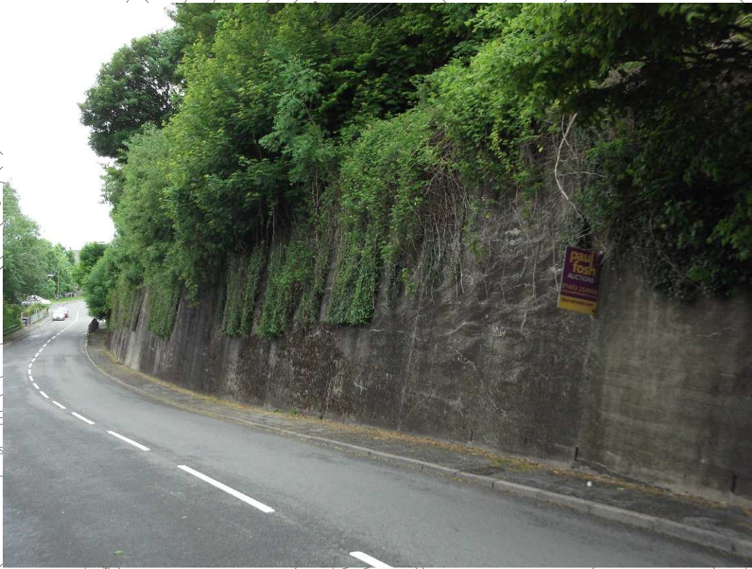
CYNFYNG ROAD RETAINING WALL (NO SIGNS OF DISTRESS)
