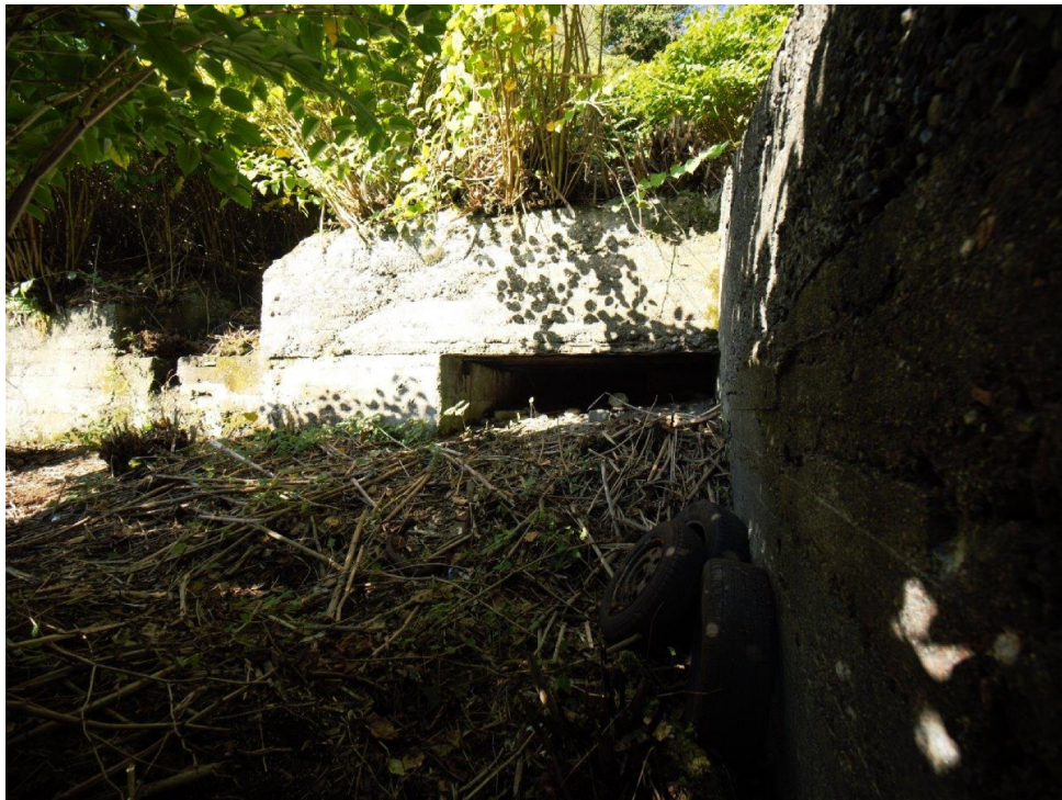
Plate 11: Possible Mine Tunnel Entry
