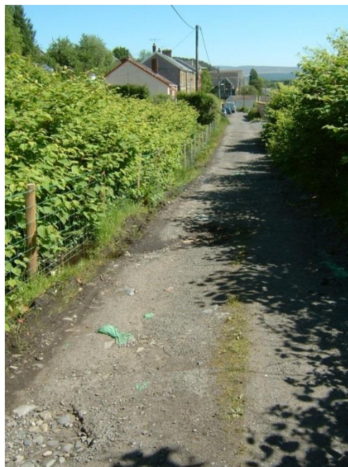
Figure 7, Photograph of Wembley Road taken on 2 nd June 2006
