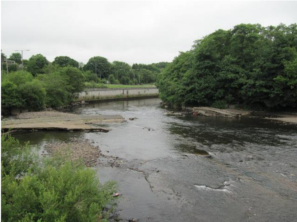
Image 1 – Weir structure at Canal Side.
