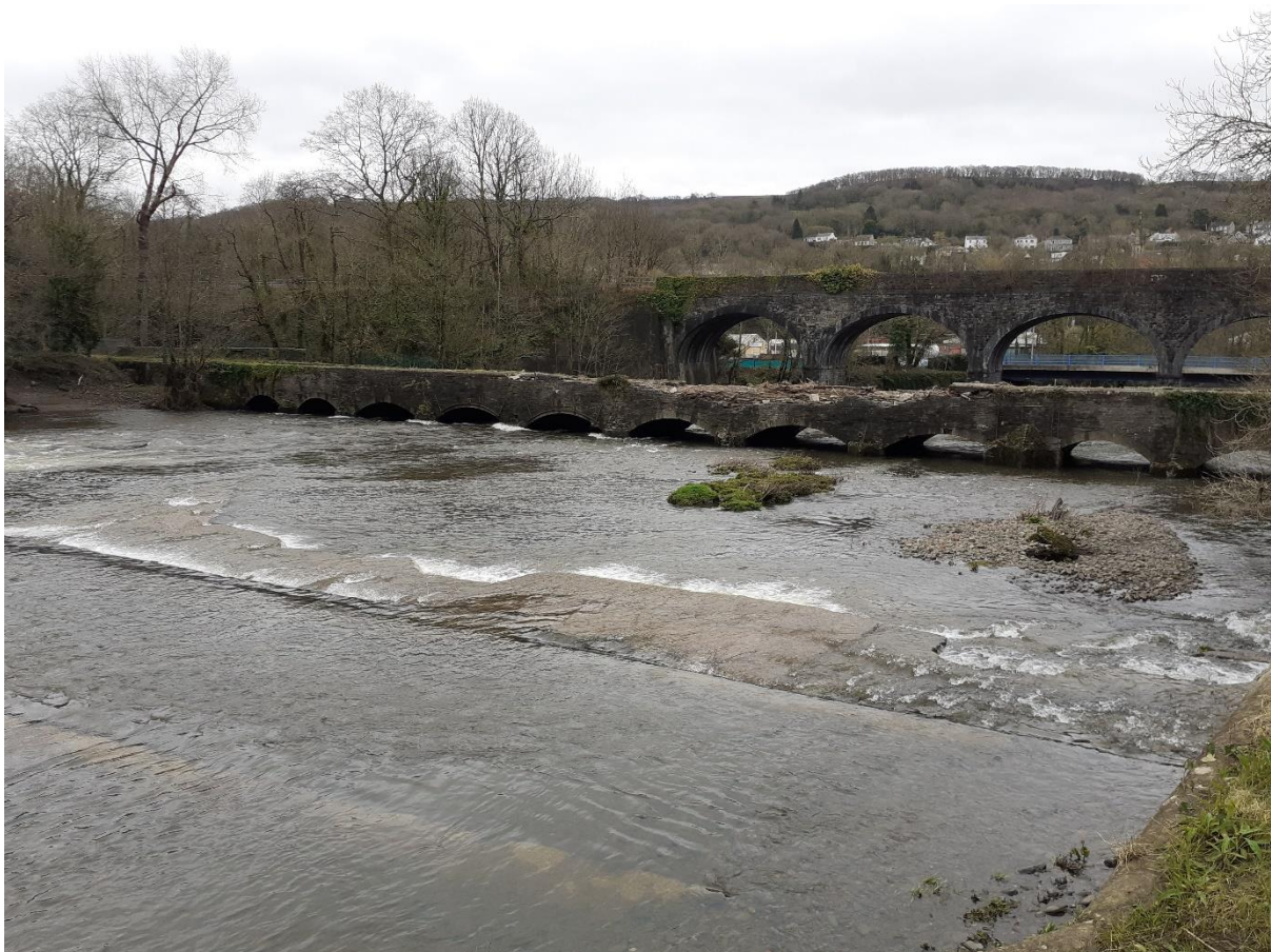
Image 2 – Tennant Canal Aqueduct
