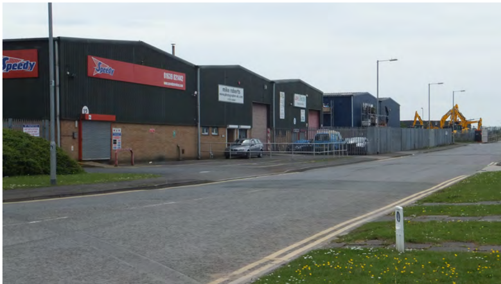
Picture 3.2 Seaway Parade Industrial Estate
