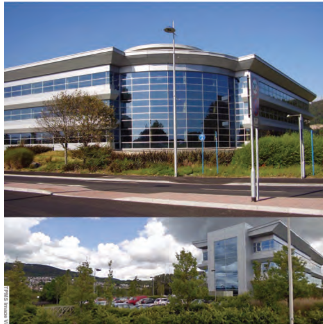
Picture 7.1 Modern Commercial Building Example
